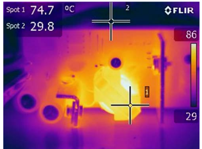
Figure 40 – 265 VAC, Full Load. Spot 1: Transformer Core. Spot 2: Ambient.
